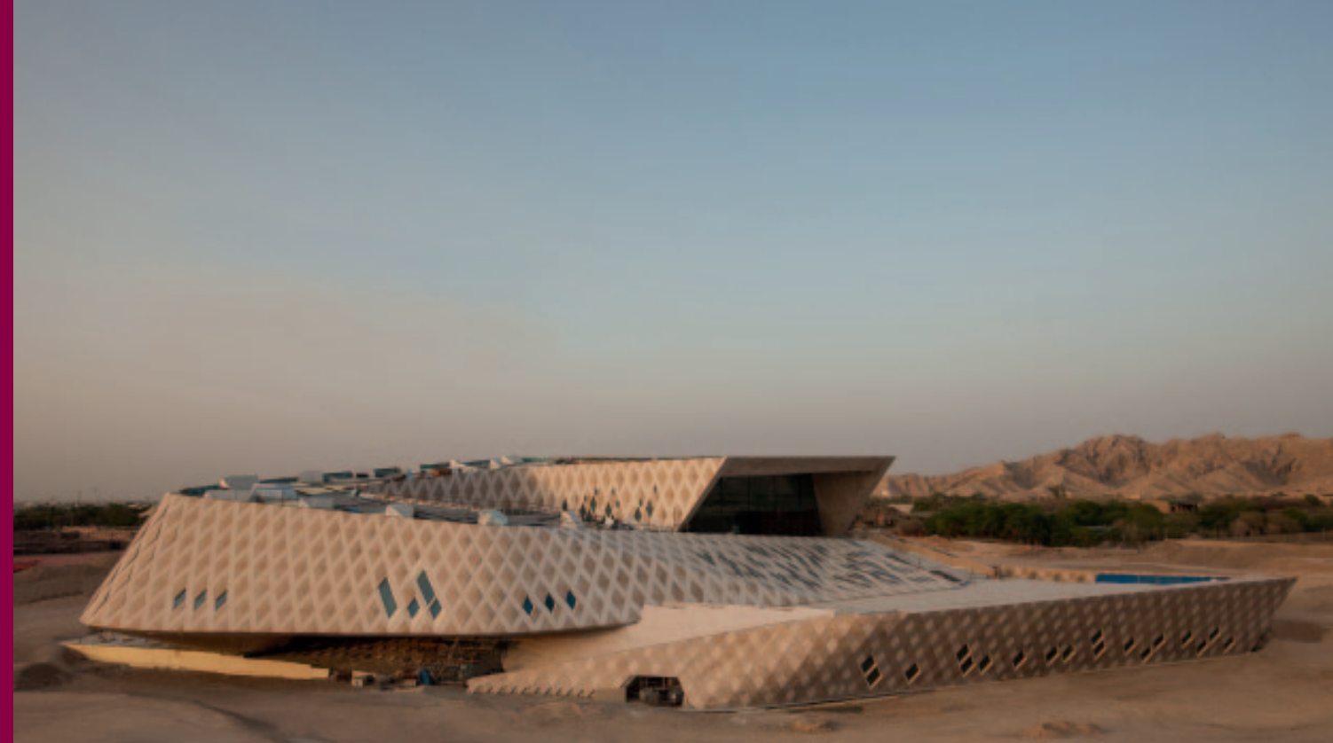
Chalabi Architekten & Partner Sheikh Zayed Desert Learning Center, Al Ain, VAE, 2013 Turn On Partner: Strabag | ED Züblin AG Foto: ED Züblin AG
